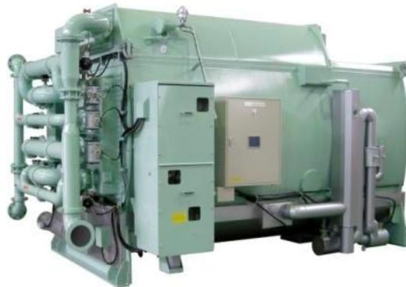
Fig.5. Adsorption chiller (Weatherite Manufacturing, UK)
