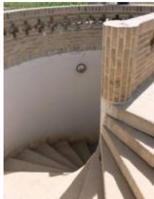
Fig. 3: Staircase of Dezful Cultural center; Ref: the author
