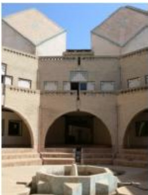
Fig. 3: Yard of Dezful Cultural Center; Ref: the author
