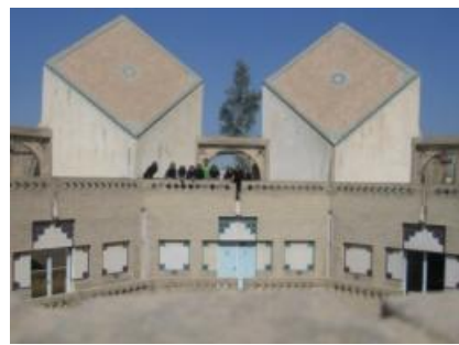
Fig. 2: Windcatchers around the yard; Dezful Cultural Center; Ref: the author
