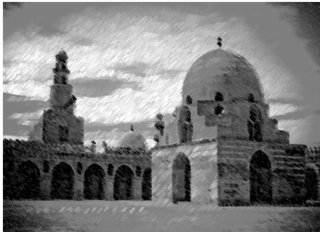
Figure 1, Ibn Toloon Mosque in Cairo, small windows in thick walls.( Illustration effects by Elbakheit A.R.)
