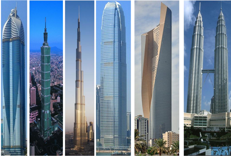
Figure 14, Rose Rayhaan, Taipei101, Burj Khalifa, Two IFC, Alhamra Firdous Tower, Petronas towers. (Courtesy of Skyscraper website).
