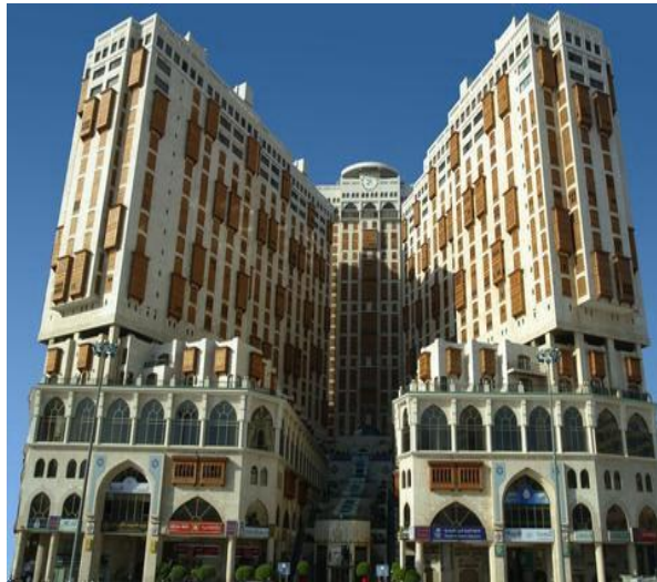
Figure 4, Mashrabiyas and wooden shutters to shade windows and provide adequate natural lighting.(Abraj-Macca tower).
